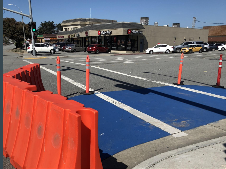
Finished Curb Extensions on Echo Ave.
